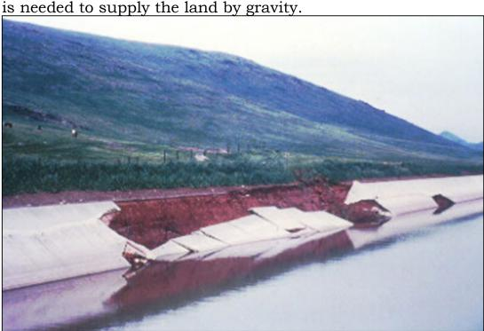
By keeping water levels high enough, erosion from rain falling in an empty earth canal is prevented.
