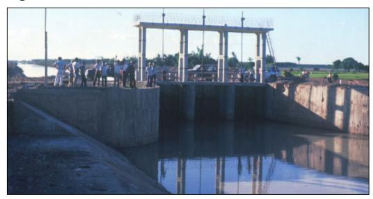
By damming a canal with cross-regulators, the water surface profile varies with the discharge from a line parallel to the canal bed at maximum flow to a horizontal line at zero flow. The volume contained between the two profiles is called the wedge volume.
